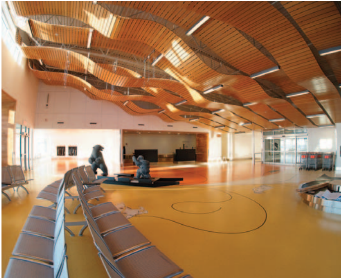
Undulating wooden suspended ceiling at Puvirnituq airport
