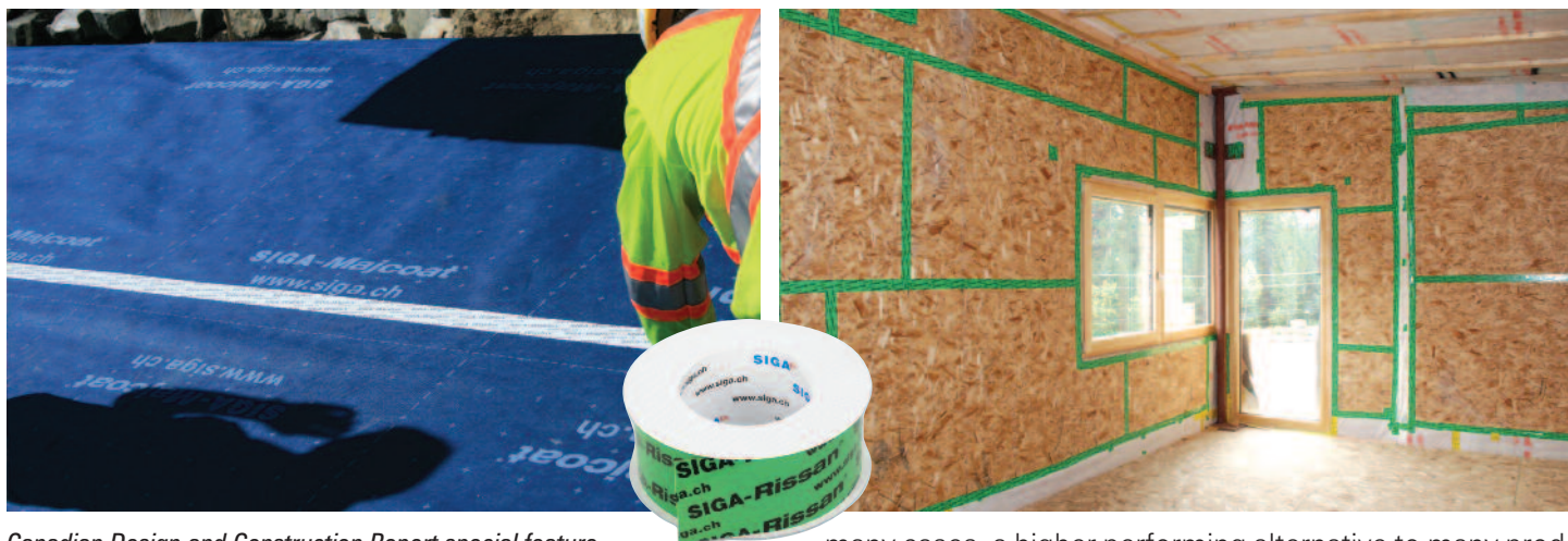
Canadian Design and Construction Report special feature
