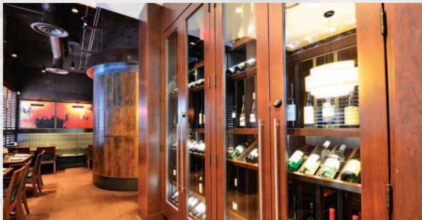
Foxwoods built and installed a complete millwork package, including a wine refrigeration unit for more than 100 bottles of wine, at the Keg Restaurant Bar and Grill in Moncton. The wall panels were built from more than 500 pieces of cherry plywood and have no visual fasteners. In some case more than 50 spread bars were used to hold a single sheet in place overnight. "What a rush," says Arseneault.
