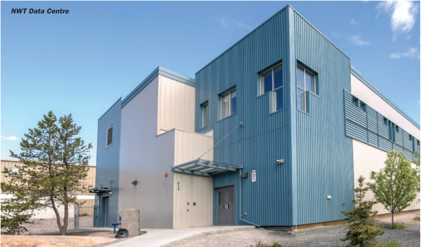
Canadian Design and Construction Report special feature
