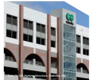
Oakville GO Parking Structure, Oakville, ON
