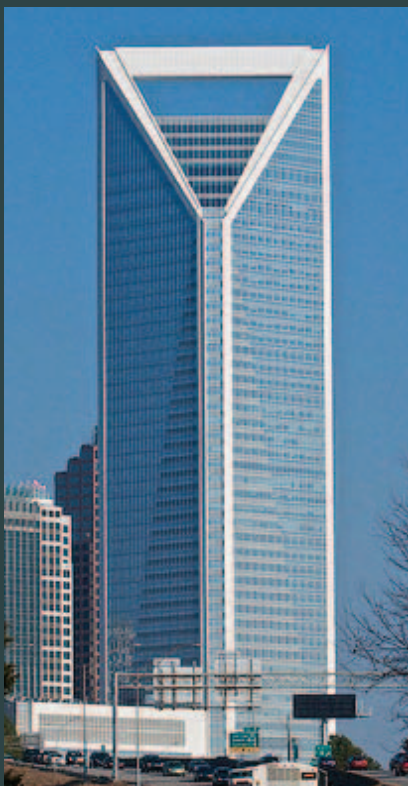
Duke Energy Building • Charlotte, NC Tallest Building in US to use double tees
