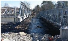
Acrow Bridge says it has supplied a single lane bridge to Nova Scotia Transportation and Infrastructure Renewal (NSTIR) for a detour during construction of a galvanized truss bridge in a neighboring location. The truss bridge is a joint project with Acrow and Canam-Bridges, a division of Canam Group Inc.
