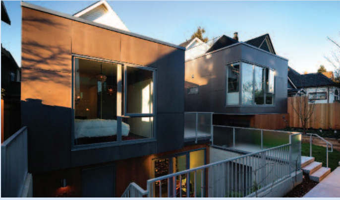
Union Street EcoHeritage (Vancouver, BC) SHAPE Architecture Inc.
