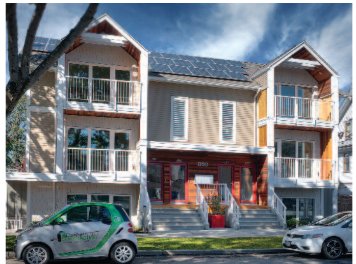
The North Park 6-unit condo is the first market condominium building in Canada to meet the stringent international Passive House standard
