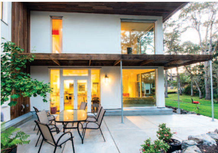
The Bernhardt Passive Home is the first Passive House built on Vancouver Island
