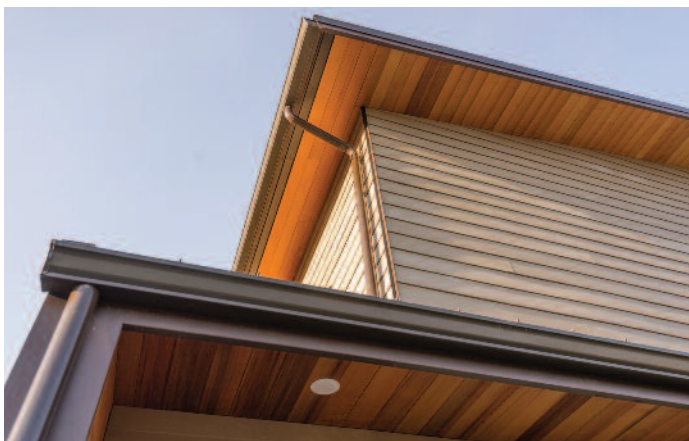
Alta Lake Passive House
