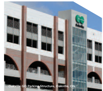
Oakville GO Parking Structure, Oakville, ON
