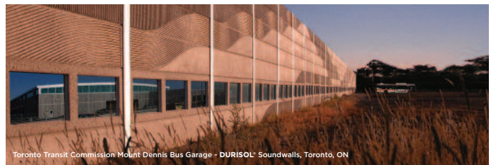
Toronto Transit Commission Molint Dennis Bus Garage - DURISOL® Soundwalls, Toronto, ON
